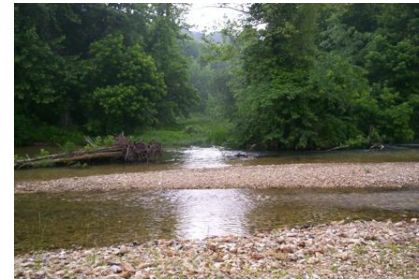
Site on Spring Creek where the new bridge is being built
